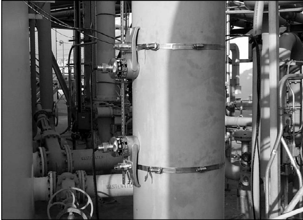
Figure 1-10: Clamp-on Ultrasonic Flow Meter (Courtesy: Endress + Hauser)
